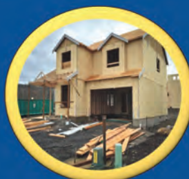
New Home Make Ready
