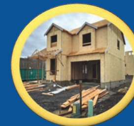
New Home Make Ready
